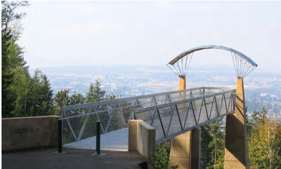
Figure 12 - Newly constructed North Viewpoint
